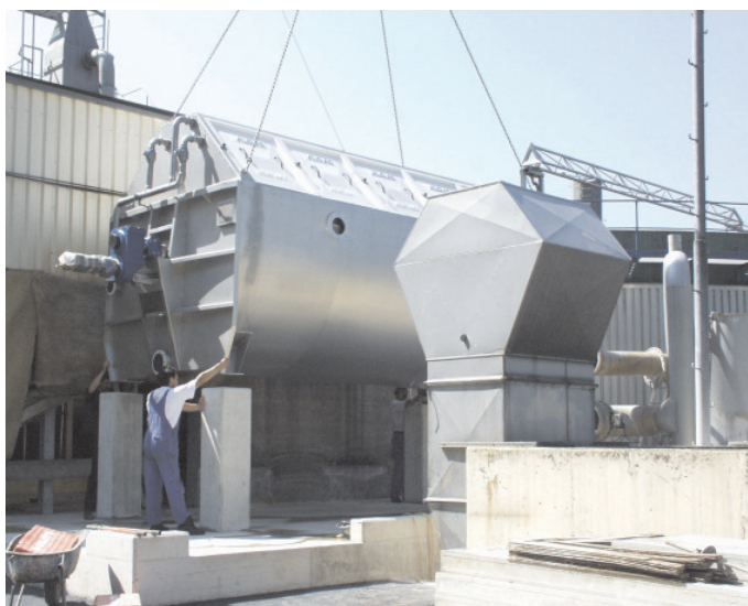
Installation of Filter
